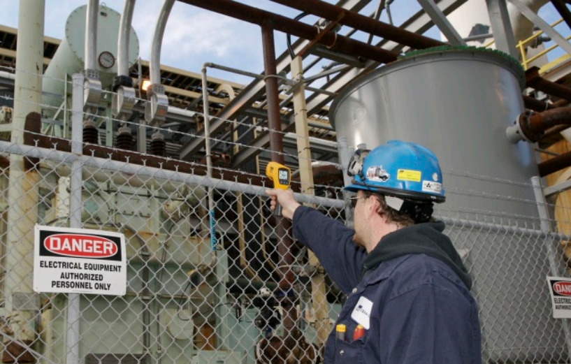
This is the 13.8 KV feeder connections to the 30 MW dc rectifier. These temperatures vary greatly, depending on ambient air and plant load.
