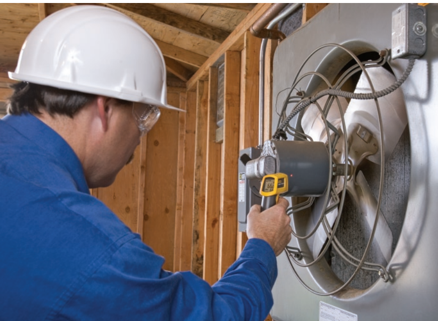
Check motor temperatures quickly, without contact.
