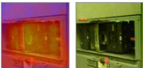
Normal operating temperature on mission critical breaker
