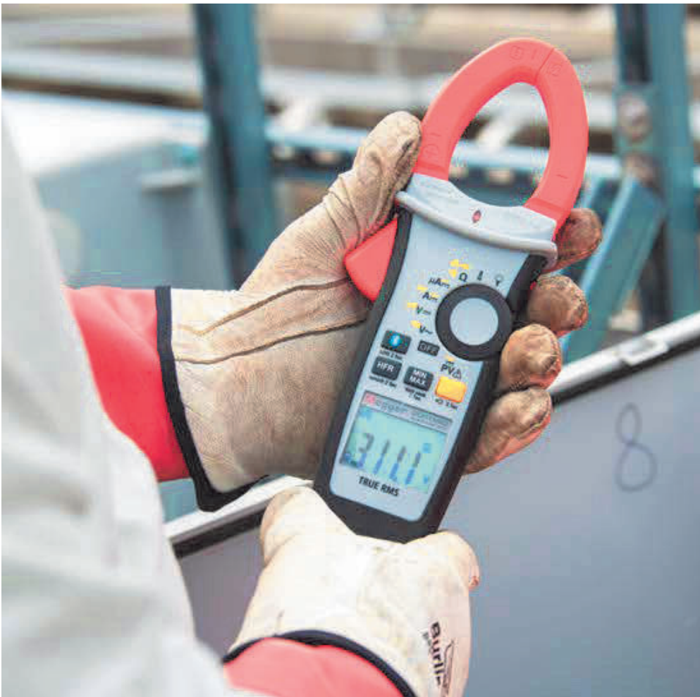
Figure 4-1: Digital multimeters are used throughout PV installation and maintenance activities.
