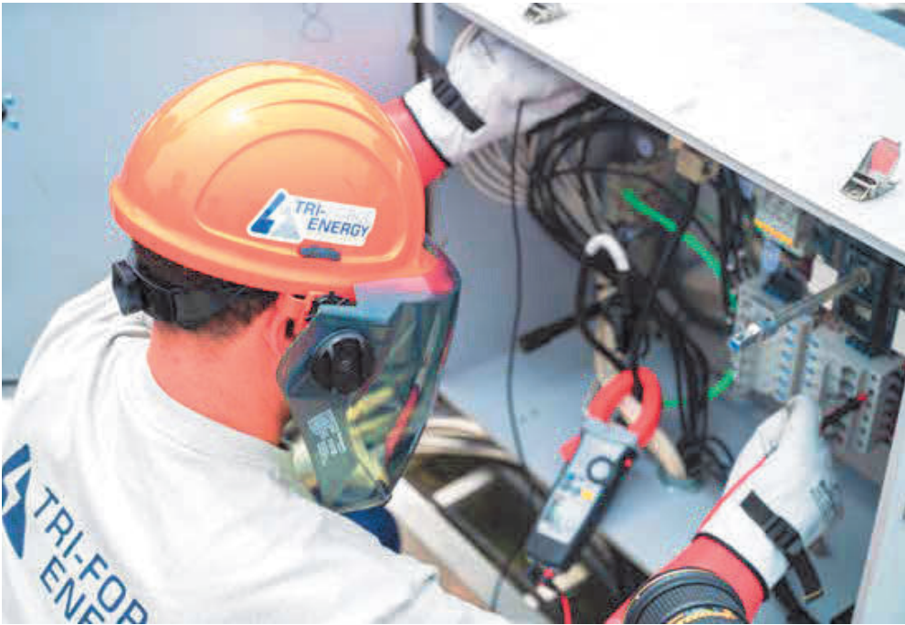
Figures 4-16 and 4-17: A field technician uses a DMM to confirm expected voltages and polarity in a PV combiner box.
