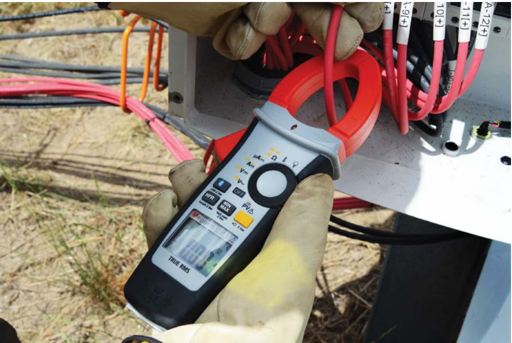
Figure 5-1: PV technicians use handheld digital multimeters to measure DC and AC circuits in PV systems.
