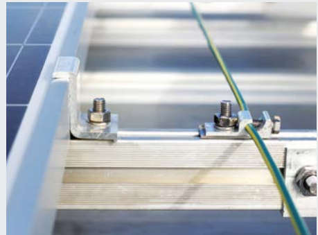
Figures 6-2 and 6-3: Left—Dubious bonding. Right—A lay-in lug bonds listed PV racking to the equipment grounding conductor.
