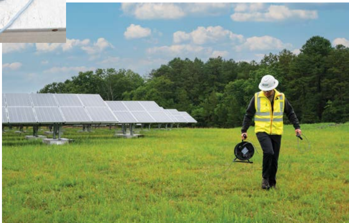
Figure 6-10: In tandem with an extension spool, the DLRO can measure electrical continuity between components up to 100 meters apart.
