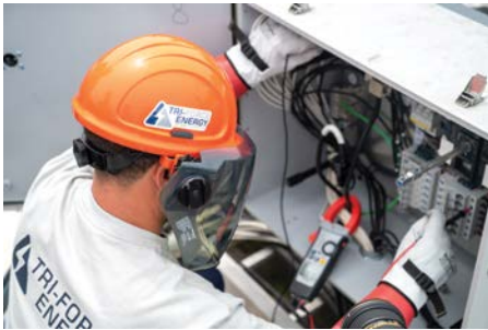
Figure 6-7: A two-point test can be performed by a single technician with a handheld DMM, but the components being tested must be within arm's reach.
